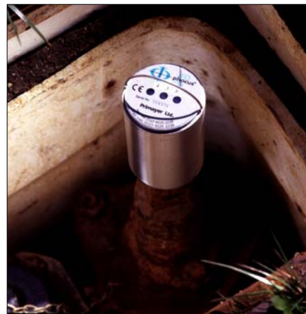
Figure 1 Phocus noise logger installation
